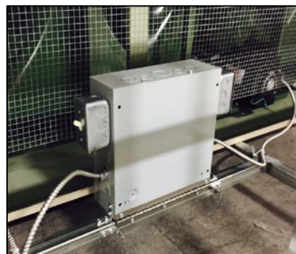
*Control Panel in Shipping Position
