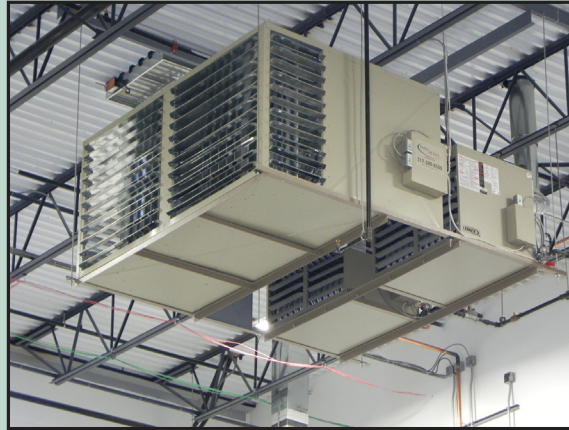
HVAC Unit The RACK ENERGY ROTATION (ER) Unit
